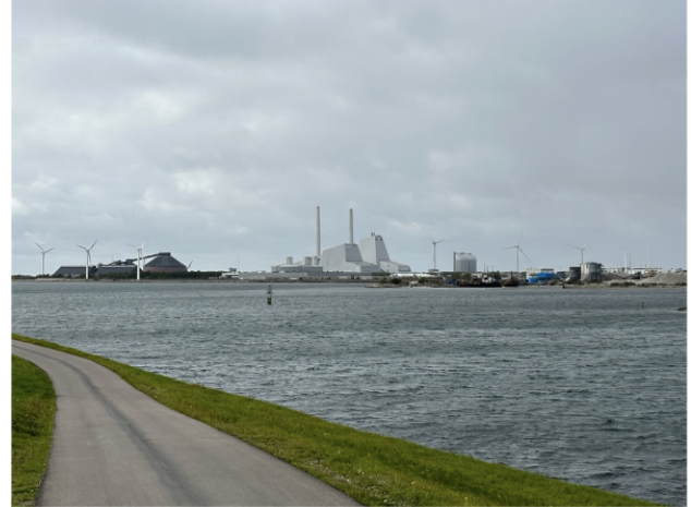
Avedøreværket, a mixed-use biomass and petroleum power plant to the south of Copenhagen with nearby wind turbines.
